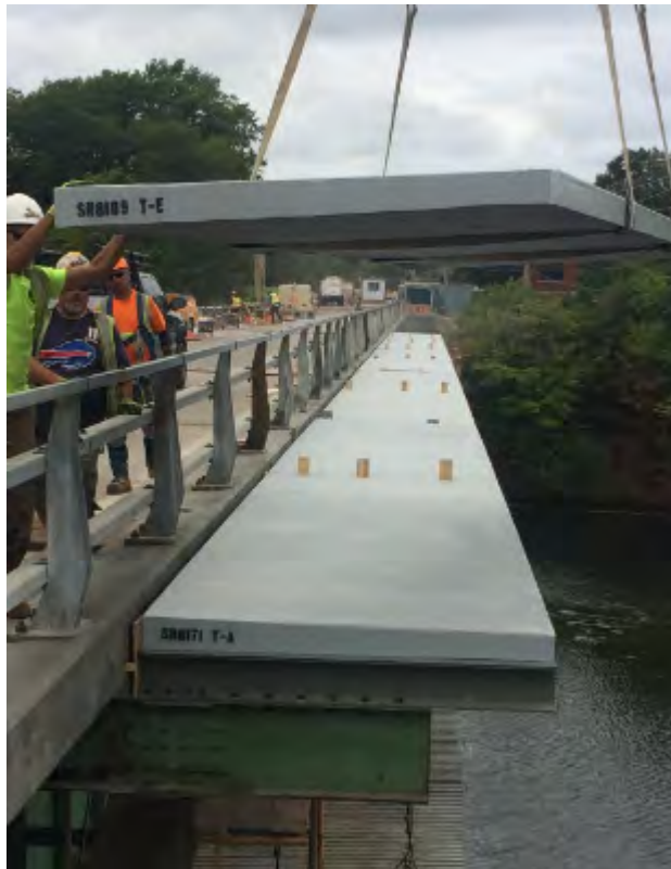
Figure 6 – Wooded shims used to set panel spacing
