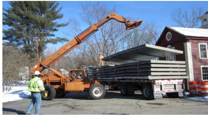
Figure 2 - Typical unloading of truck
