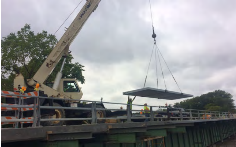
Figure 5 – Panel installation
