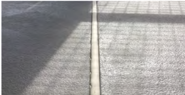
Figure 9 – Colorseal System Installed Between Two Panels
