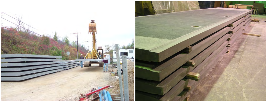
Figures 3 &amp; 4 – Stacking of panels on site
