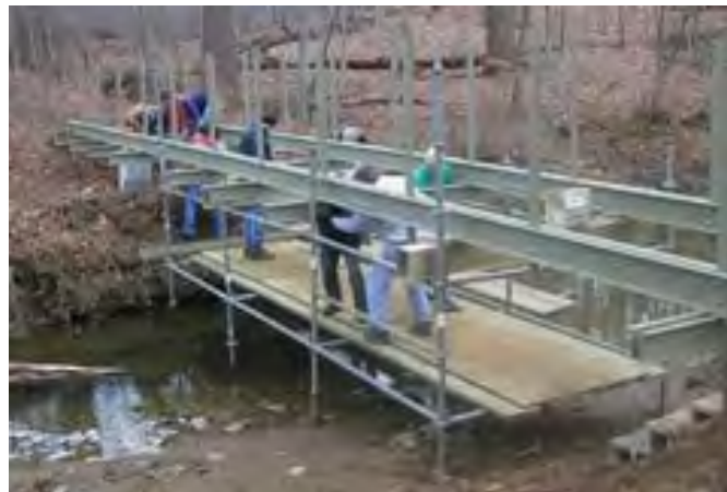
Figure 7 – Scaffolding being used as a support
