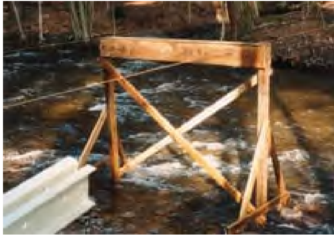
Figure 6 – Temporary support in streambed
