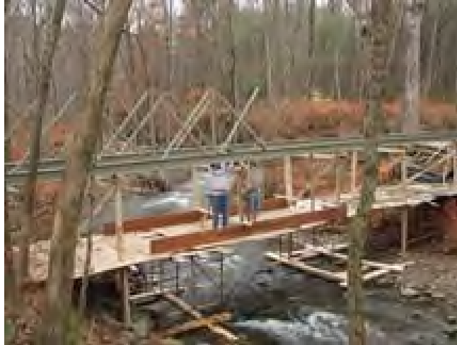
Figure 8 – Scaffolding and lumber being used as a support
