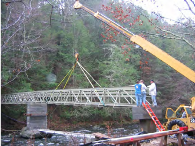
Figure 10 – Crane lifting bridge into place
