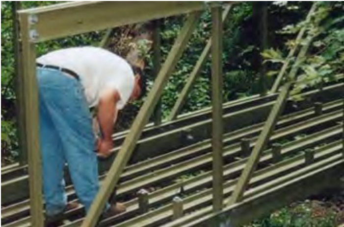
Figure 5 – Trusses being connected
