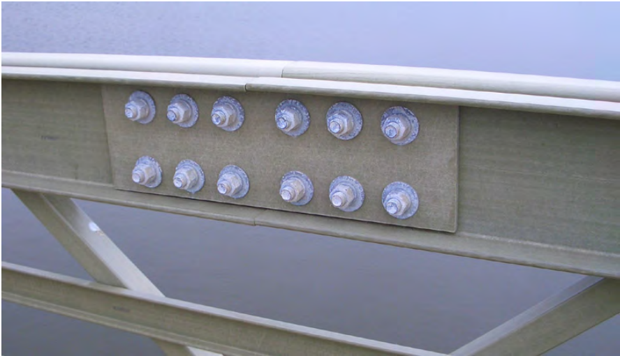
Figure 11 – Bridge Splice
