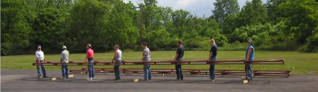
Figure 3 – Truss being lifted by crew
