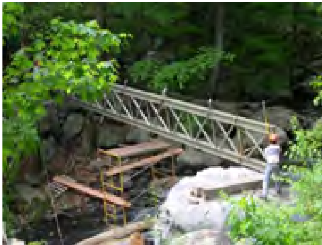
Figure 9 – Bridge truss being pulled across using a high line
