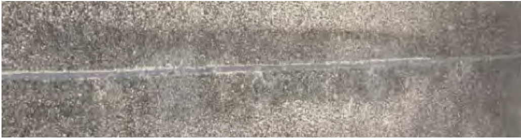
Figure 12 – LM Joint Filler Installed Between Two Panels
