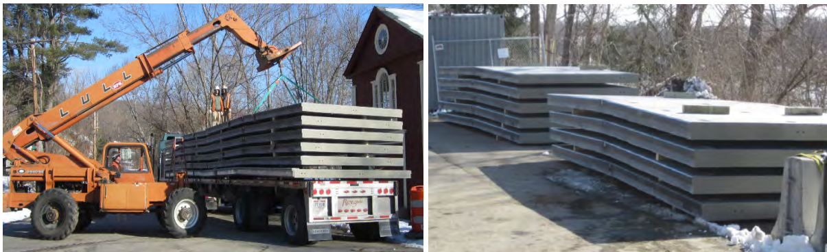
Figures 4 & 5 – Unloading and Stacking of panels on site
