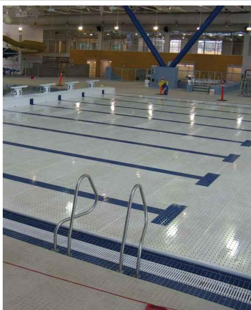
LEFT: PHOTO COURTESY OF PRECISION FIBRE STRUCTURES CENTER: PHOTO COURTESY OF CLEVELAND BRIDGE
