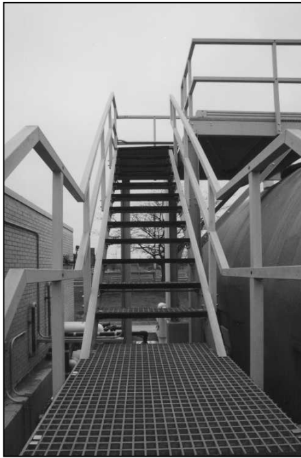
Fiberglass platform systems are ideal in highly corrosive areas.
