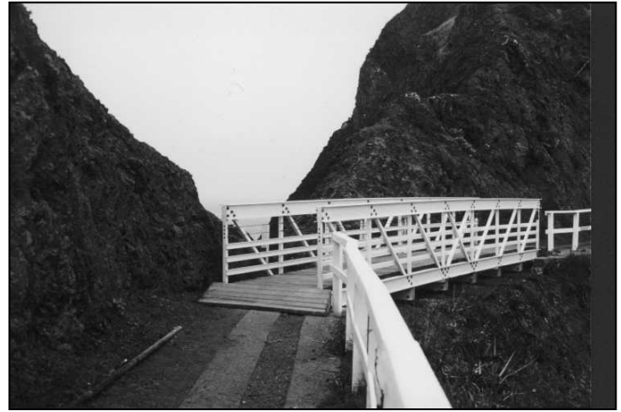
Bridges are easily installed in hard-to-access areas.
