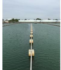
spans to minimize structural framing and corrosion resistant for long service life. The options at that time were redwood baffle planks, with their associated environmental concerns, and conventional fiberglass panels. The products were required to be third party certified to NSF standards for processing of potable water.
