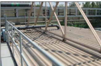
*Tuff Span truss-supported cover*
