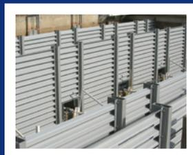
*FRP Structural Baffle Wall*
