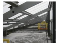
For walk-in access or as a UV and debris barrier, Enduro Tuff Span tank covers offer a cost effective, corrosion resistant, structural enclosure. For more information and details on the Tuff Span cover, please visit page 17.
