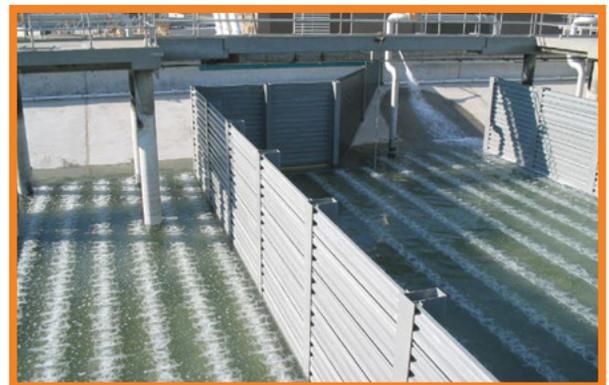
Enduro FRP SlideGuide "H" baffle series in aeration basin
