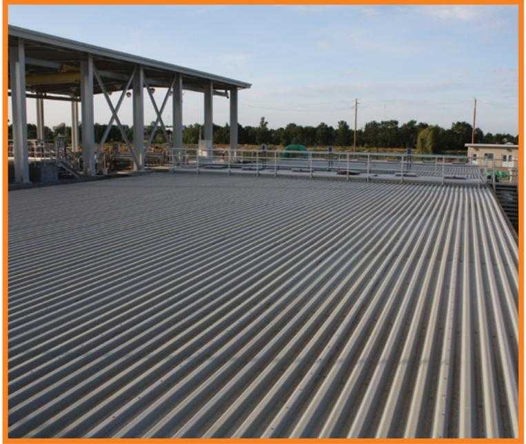
*Tuff Span low-profile tank cover system with FRP beams
