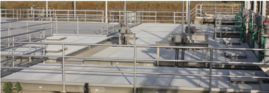
XL6 clear span tank cover system with access hatches UV Disinfection Process
