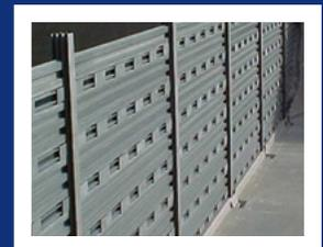
*Perforated Baffle Wall*
