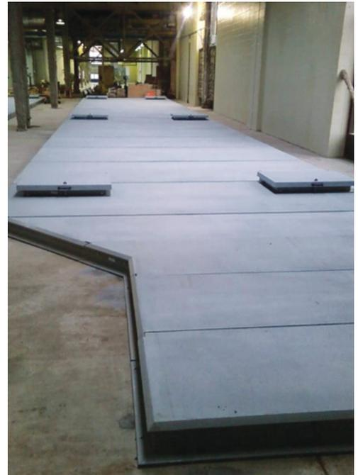
XL6 clear span tank cover system with angle cut panels and access hatches over filtrate storage tanks
