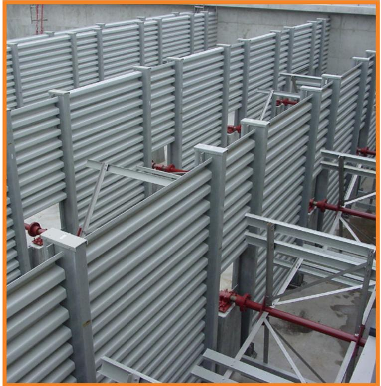
Flocculation Baffle Walls using Enduro Baffle D
