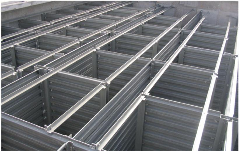
Enduro "D" & "H" baffle wall systems with top-braced FRP columns
