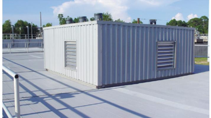
Tuff Span removable enclosure with FRP panels, beams and louvers over floating aerator. Beam-supported cover - Aeration Basin
