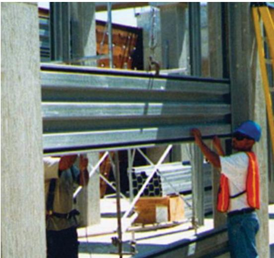
"H" series baffle panels are stacked from basin bottom to top and do not require fastening to supports.
