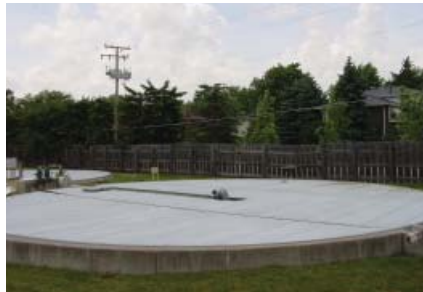
XL6 beam-supported tank cover system 50' Diameter Clarifier
