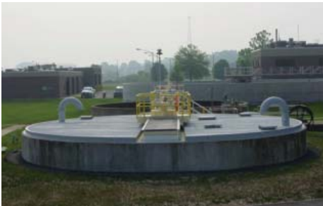
XL6 clear span tank cover with access hatches & vents 40' Diameter Sludge Thickener Cover
