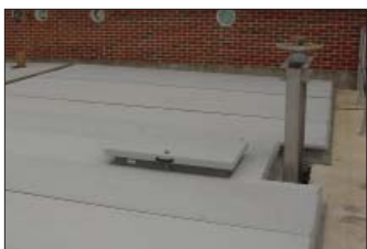
Shop-fabricated panels include notched openings & self-contained access hatches.
