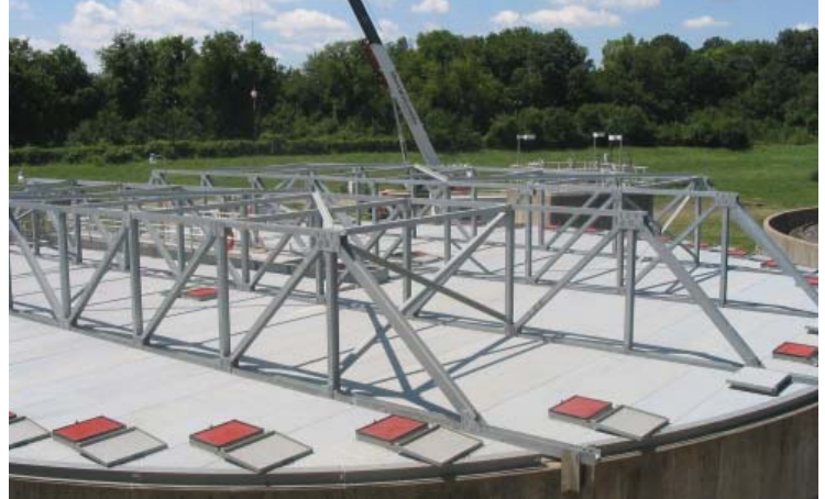
XL6 truss-supported tank cover system with FRP access hatches and safety grating 88' Diameter Gravity Thickener
