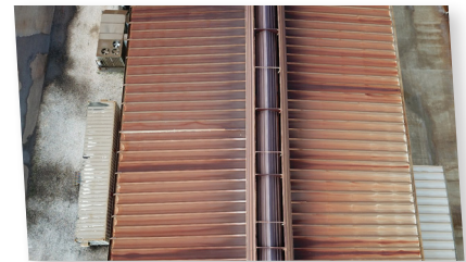
BEFORE ENDURO PANEL INSTALLATION
