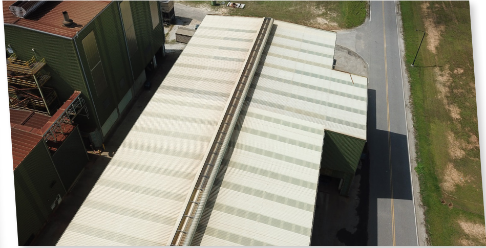
NEW ENDURO PANEL INSTALLATION
