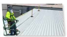
shop applied acrylic polymer coating. Translucent white panels were chosen providing an aesthetically pleasing appearance while increasing natural light under the canopy. These noted benefits of Tuff Span™ will provide a long−term, structurally performing canopy system.
