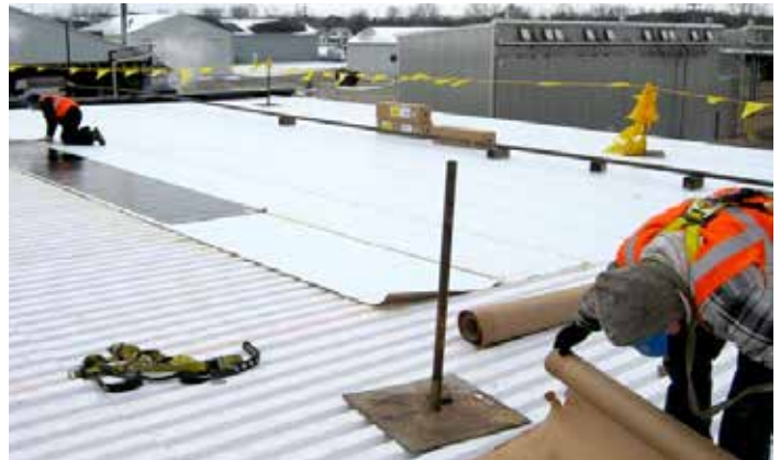
Mechanical fasteners, hot or cold adhesives can be used to attach roofing membrane and insulation.
