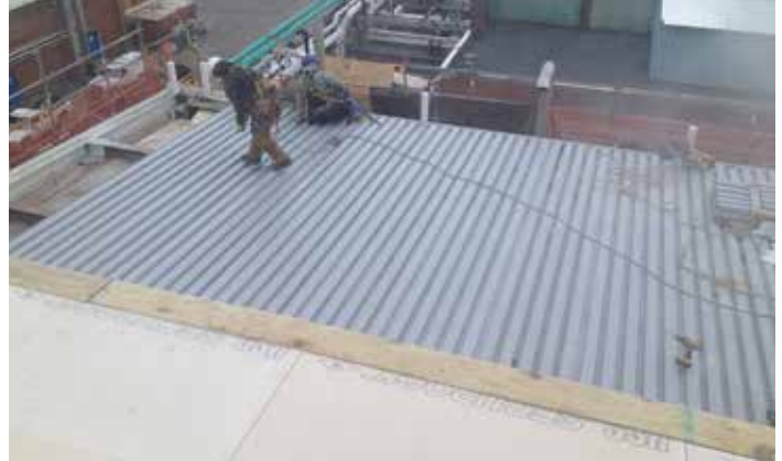
Corrosion resistant Tuff Span is a suitable substrate for either single-ply or built-up roofing.
