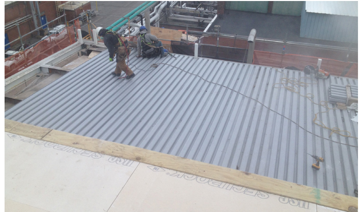
Tuff Span Roof Deck Installation at Chemical Plant
