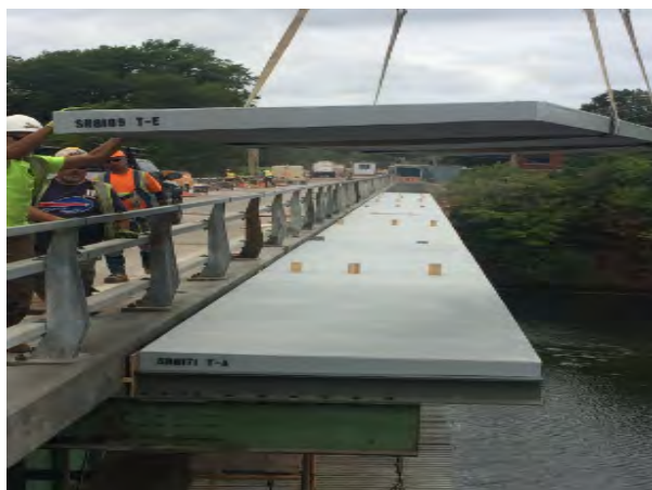
Figure 5 – Wood Shims Used to Set Panel Spacing
