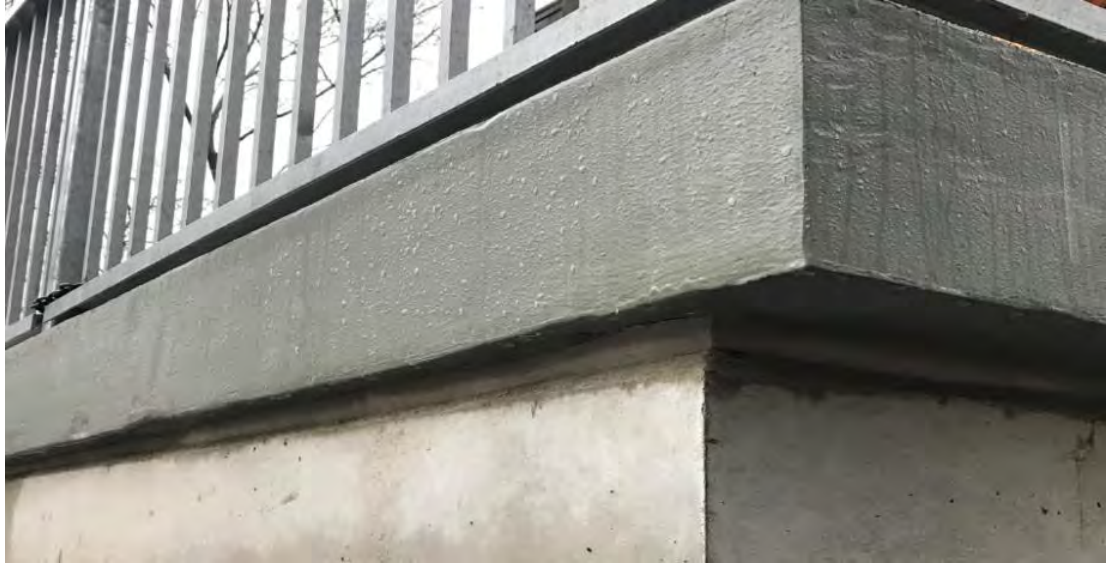
Figure 8 – Finished Grout Pad Below Panel
