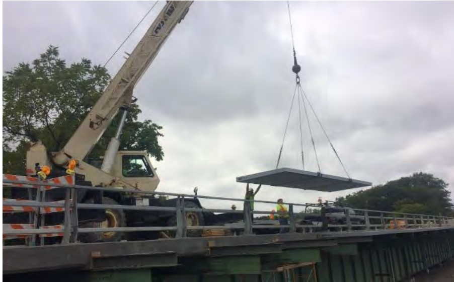
Figure 4 – Panel Installation
