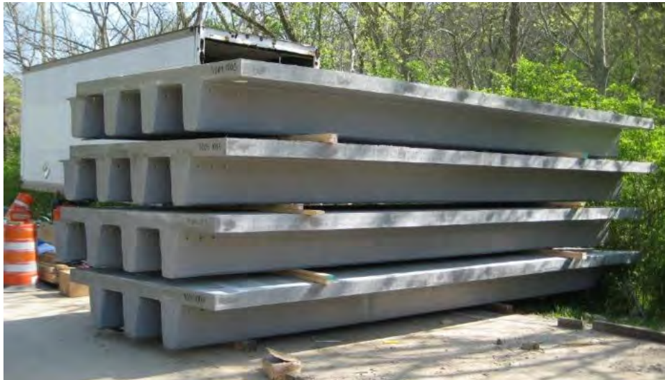
Figure 3 – Stacking of Panels on Site
