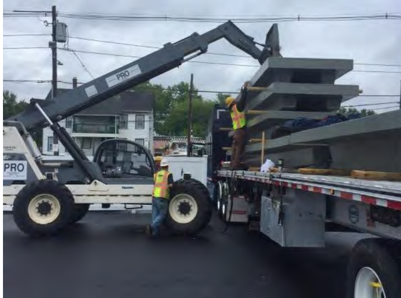
Figure 2 - Typical Truck Loading
