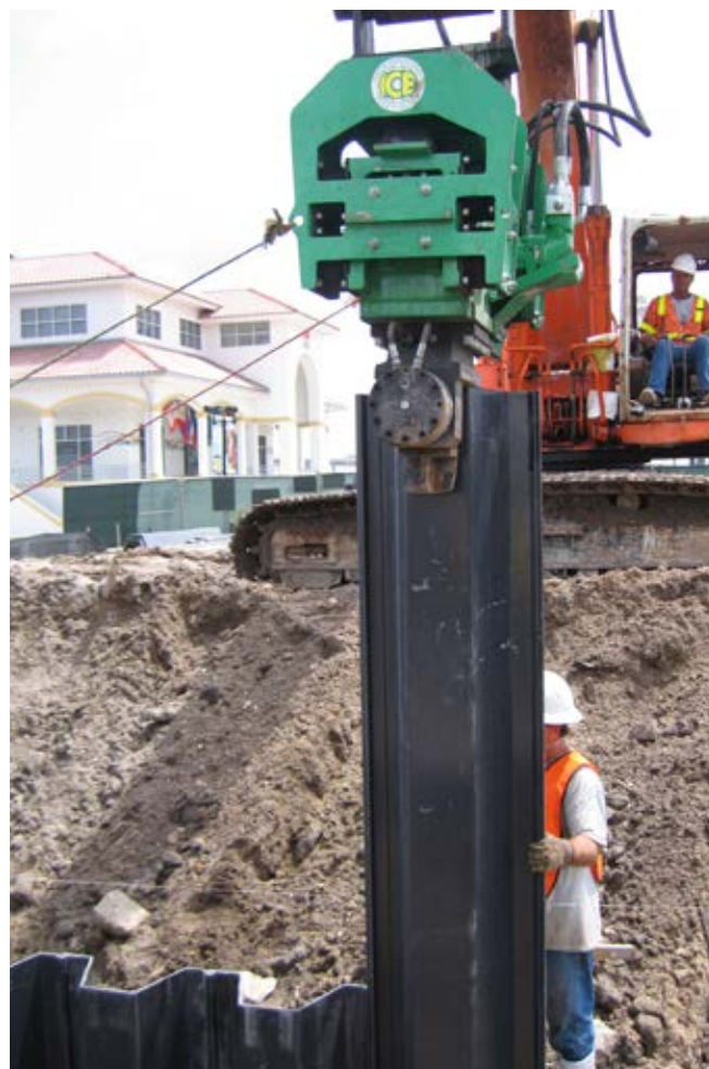
Vibratory Hammer Installation Example
