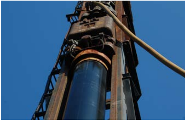
Vulcan 01 Impact Hammer Driving 16” Diameter Pile
