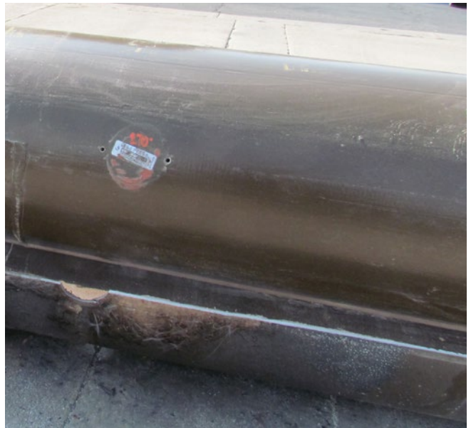
The uncompromised FRP pole after the charred outer sleeve has been removed post-fire.
