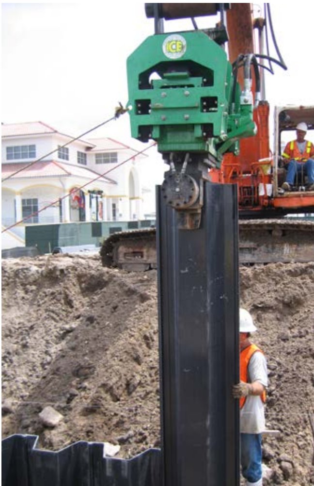
Vibratory Hammer Installation Example
