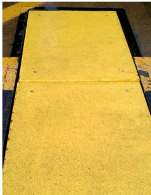
FRP Covers, in use at Naval Station Norfolk, at 170 lb each
