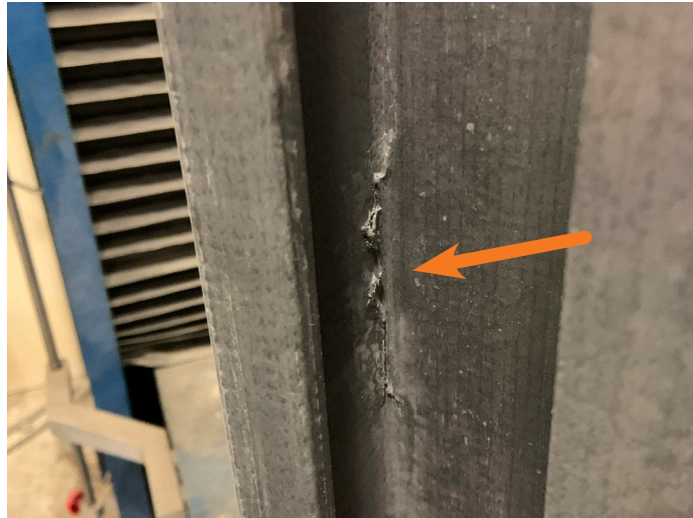
Figure 6: Two-foot span shear failure
