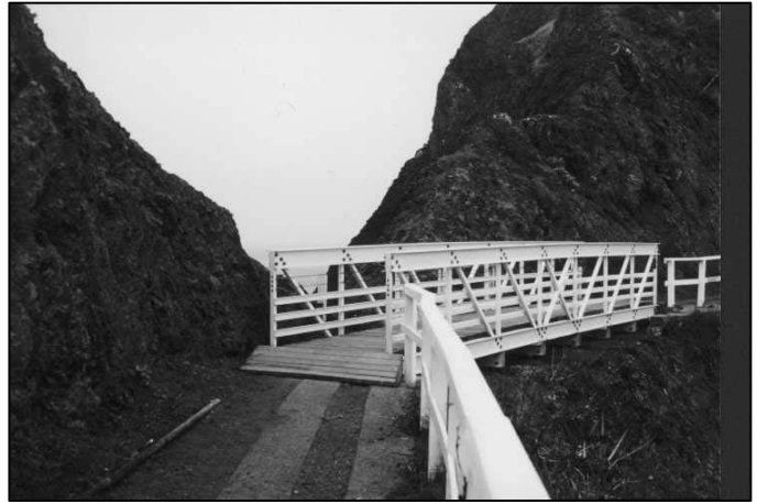
Bridges are easily installed in hard-to-access areas.
