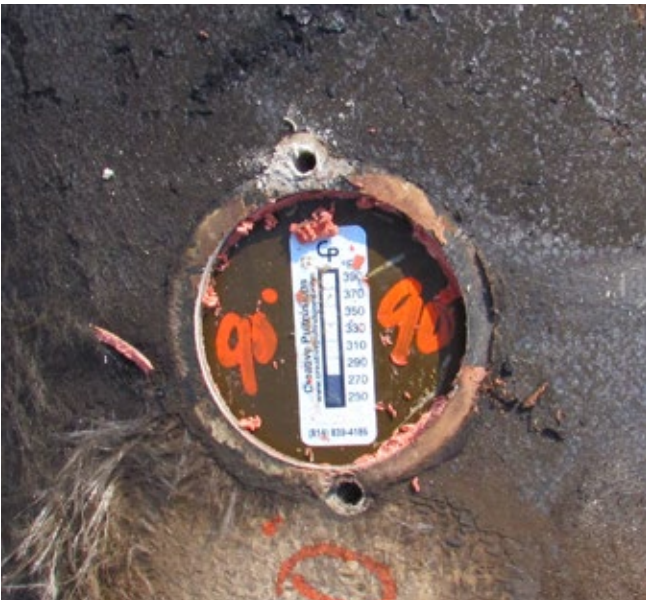
Irreversible Temperature Measuring Device after fire exposure, viewed through the fire protection sleeve.
