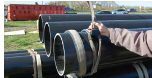
Lift-It Sling Double Wrapped Around the Pile
