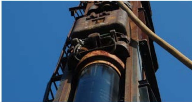
Vulcan 01 Impact Hammer Driving 16" Diameter Pile
